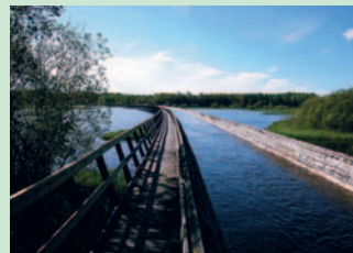
The Timber flume
